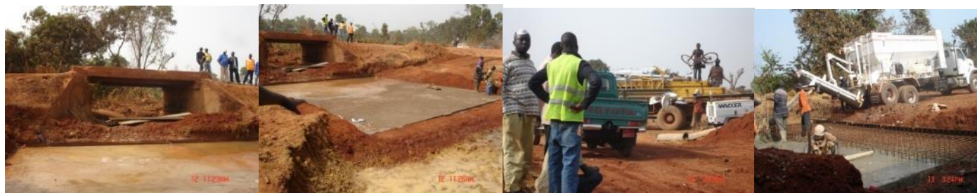
BITUMAGE ROUTES HAUTE GUINEE
