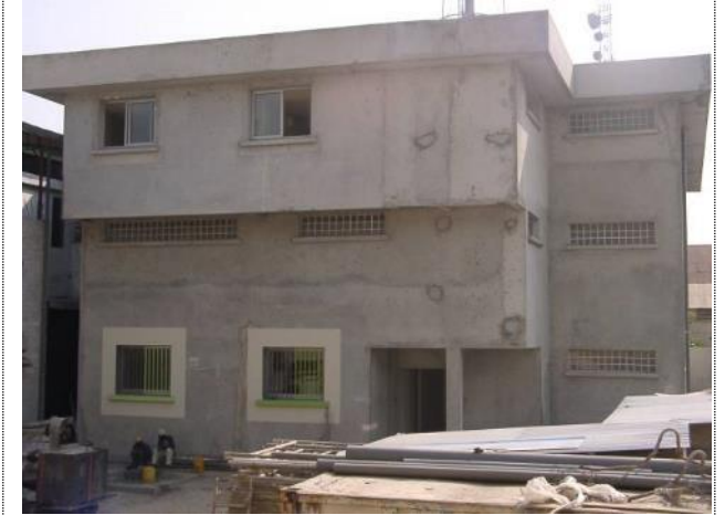
BATIMENT TECHNIQUE INTERCEL KALOUM CONAKRY
